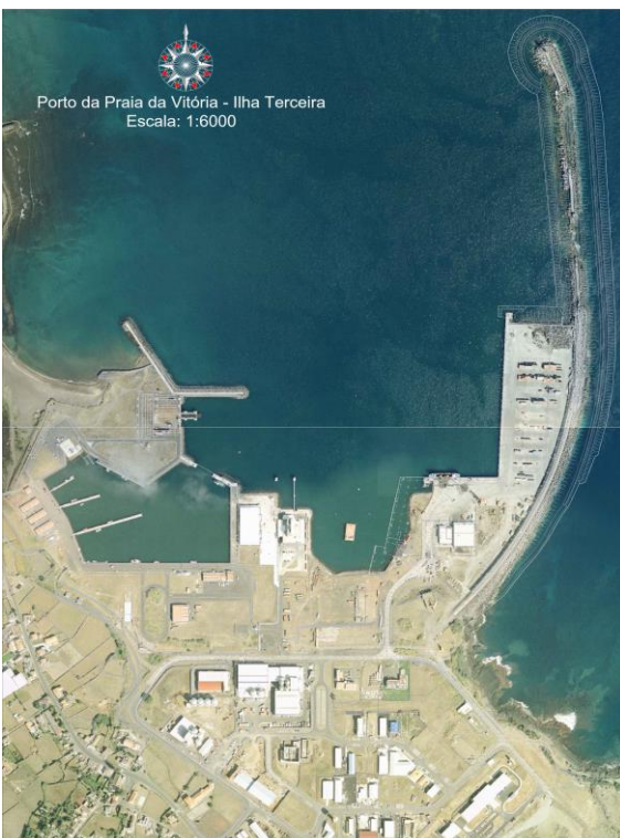
Image 3: Praia da Vitória Harbour Basin Plant – Terceira Island.
