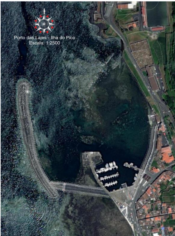
Image 9: Lajes Harbour Basin Plant – Pico Island.
